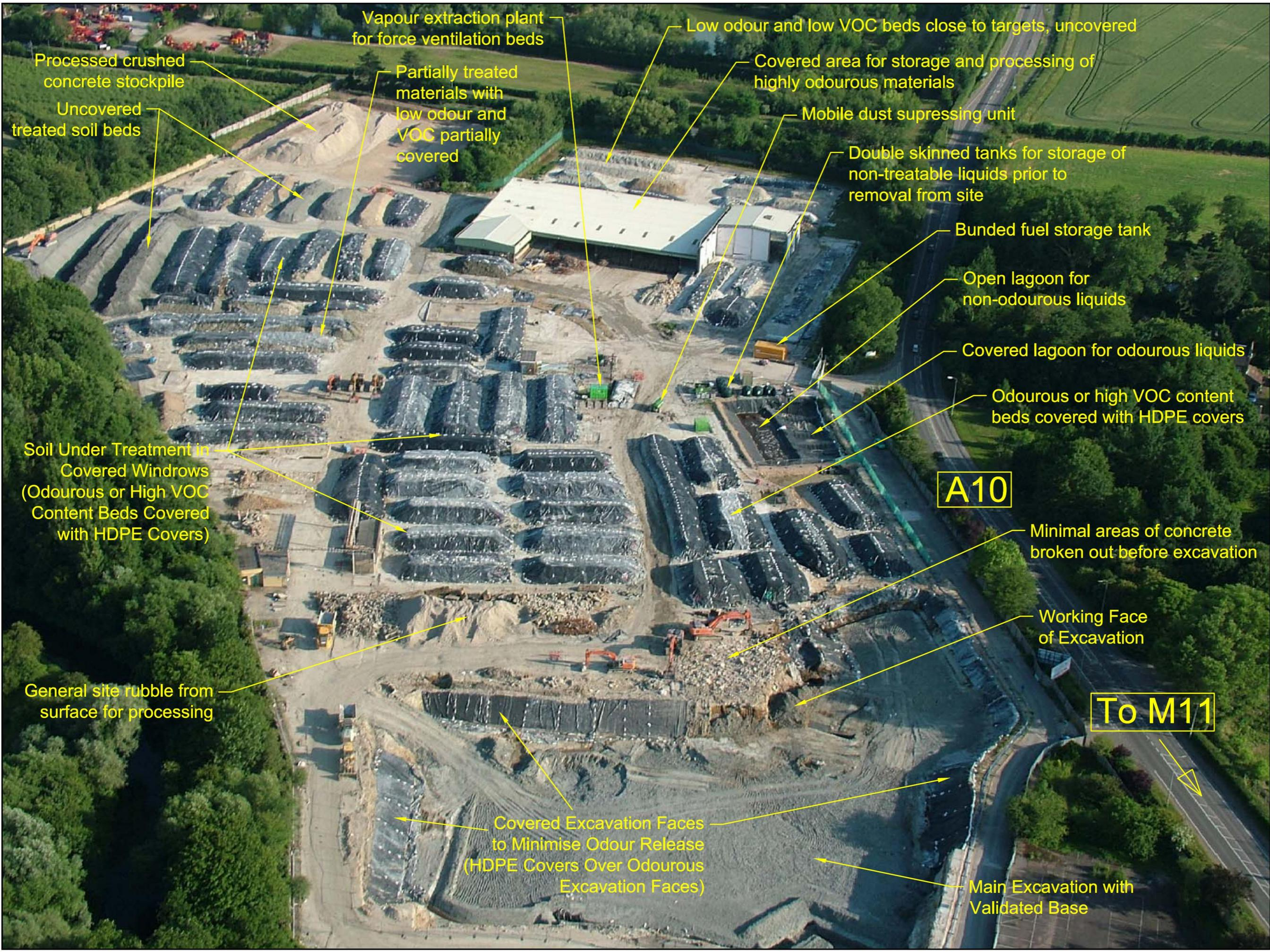
Vapour extraction plant for force ventilation beds
